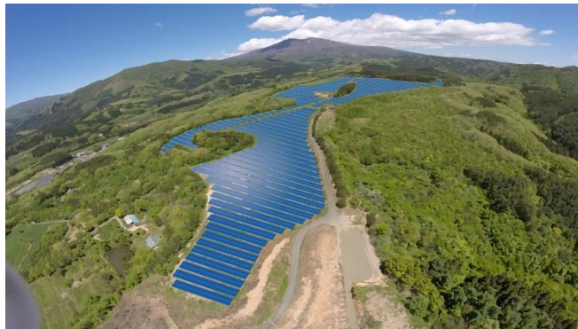
Rendering of completed mega-solar project currently under construction in Shichikashuku Town, Miyagi Prefecture
